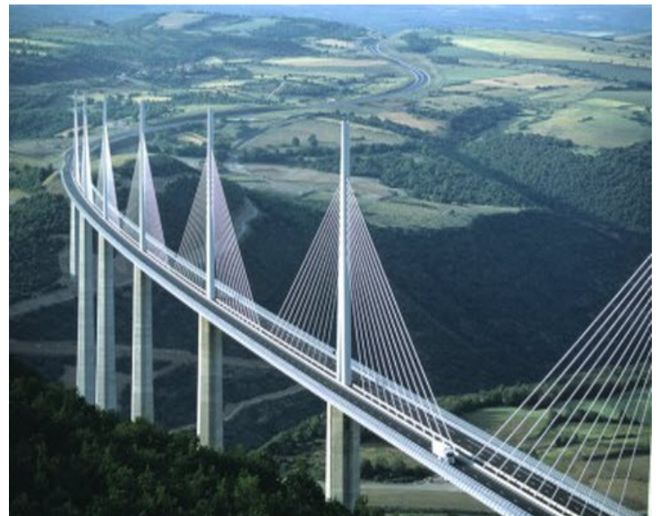
Milau Viaduct Bridge: An Engineering Marvel, the bridge connects the motorway from Paris to Barcelona. Each of its sections span 350 m in length and some of its columns are even higher than the Eiffel Tower
